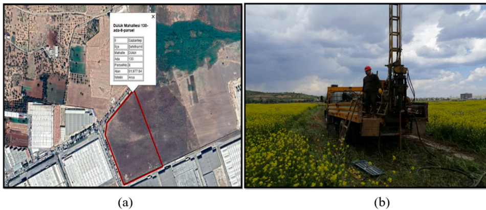
Fig. 4. (a) Location of construction SC column;(b) Grout machine.
