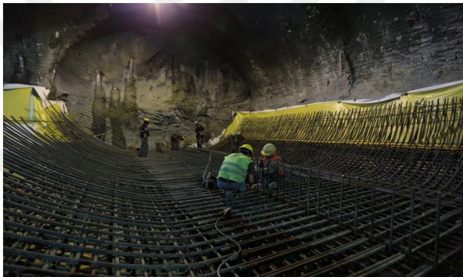
Figure 7.14 Site Manufacturing Photos of NATM Construction Method
