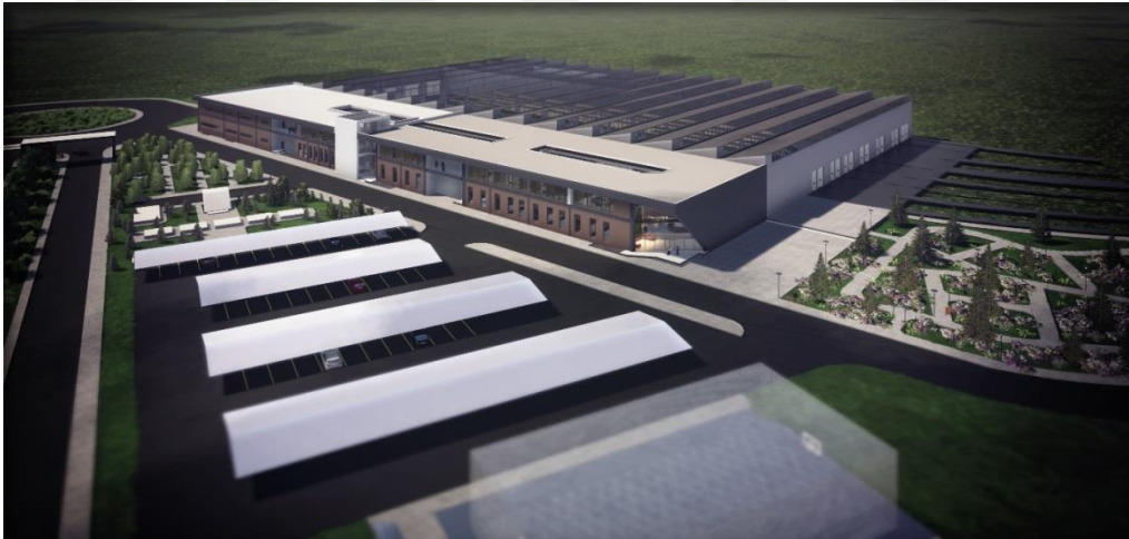
Figure 5.39 Warehouse Area General View
