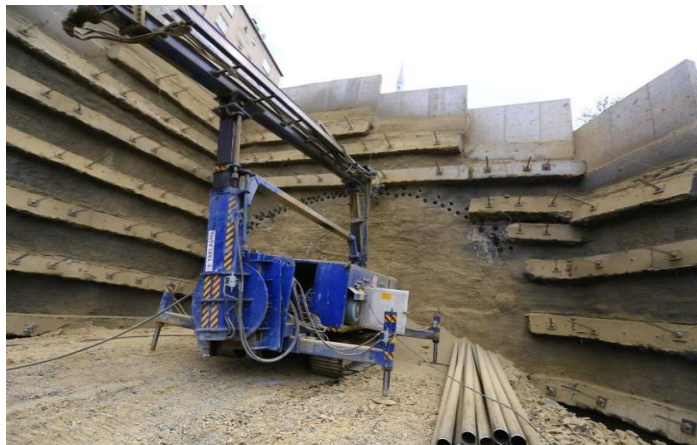
Figure 7.13 Lower half shotcrete and fortification fabrication
