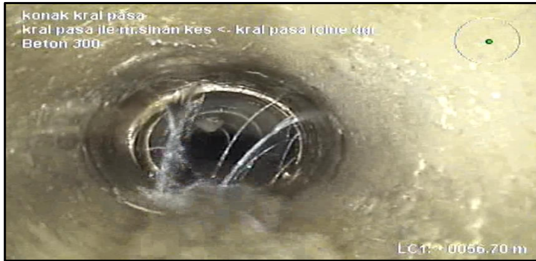
Figure 5.5. A Water Loss Detected During Channel Imaging
