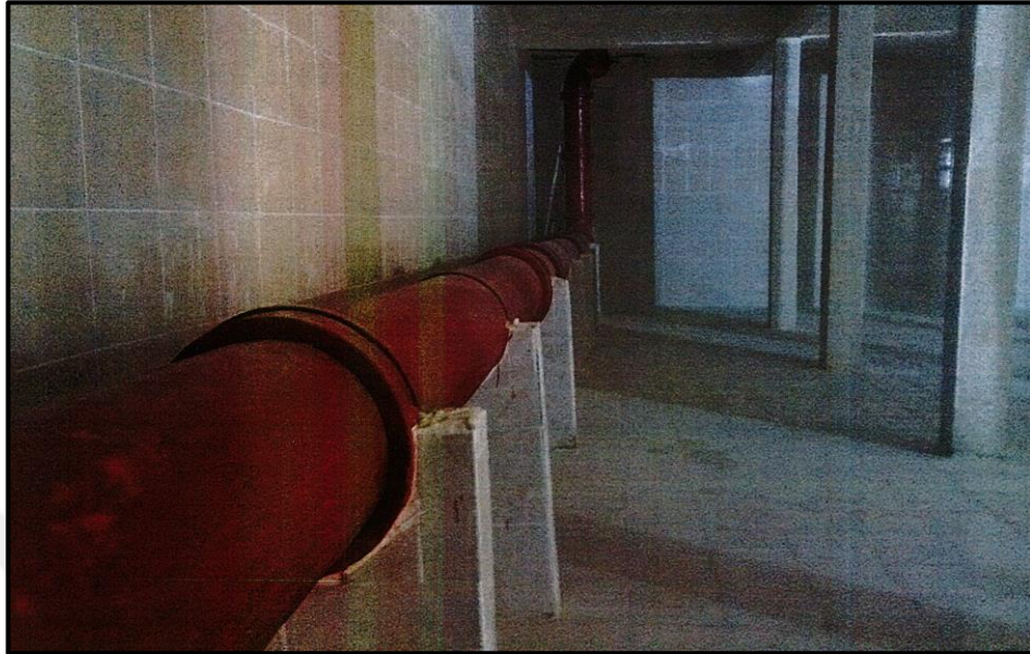
Figure 5.7. Renewal of Water Storage Tanks
