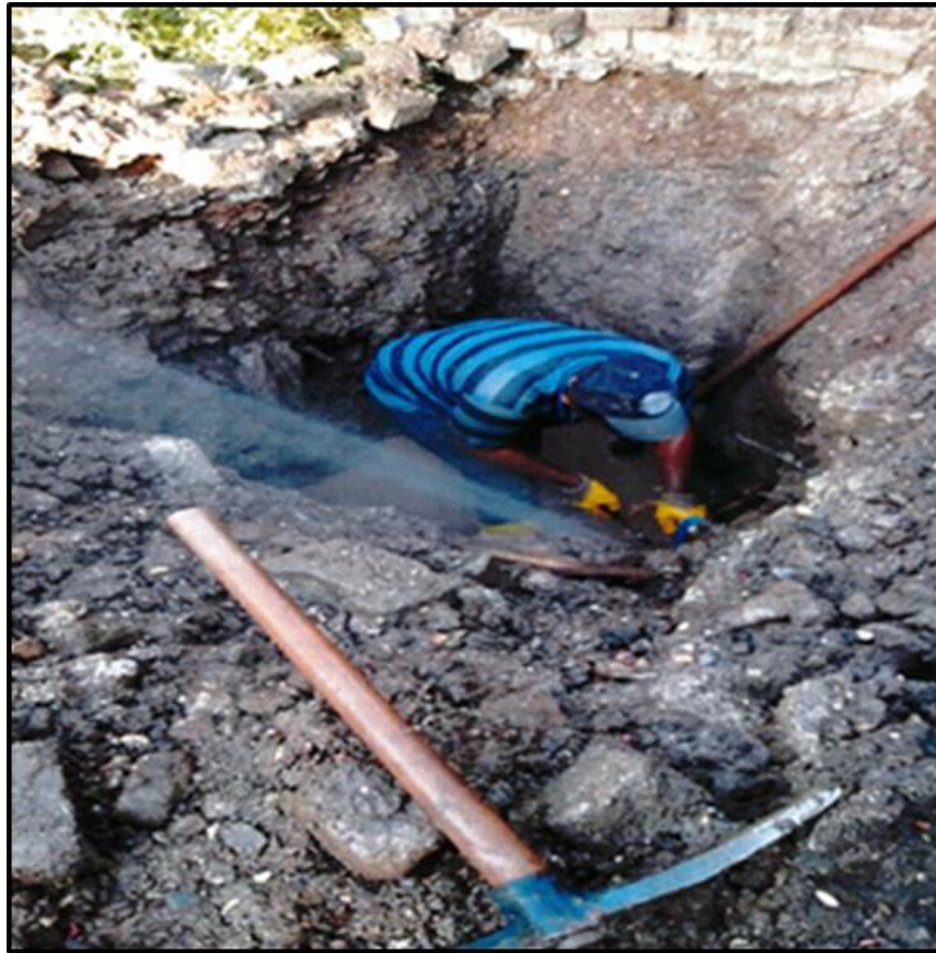
Figure 2.6. Example about Physical Water Losses
