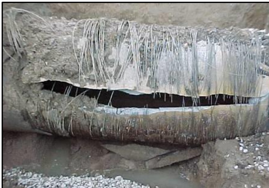
Figure 5.6. An Old Prestressed Concrete Pipe
