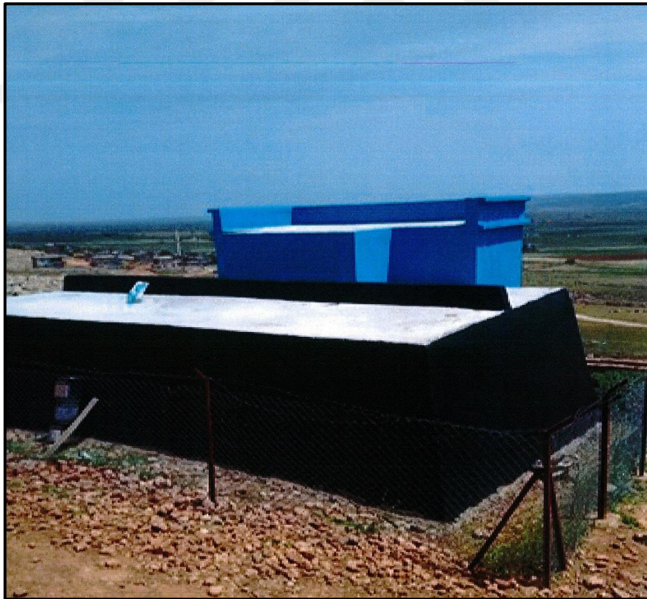
Figure A.4. Renewal of Water Storage Tanks
