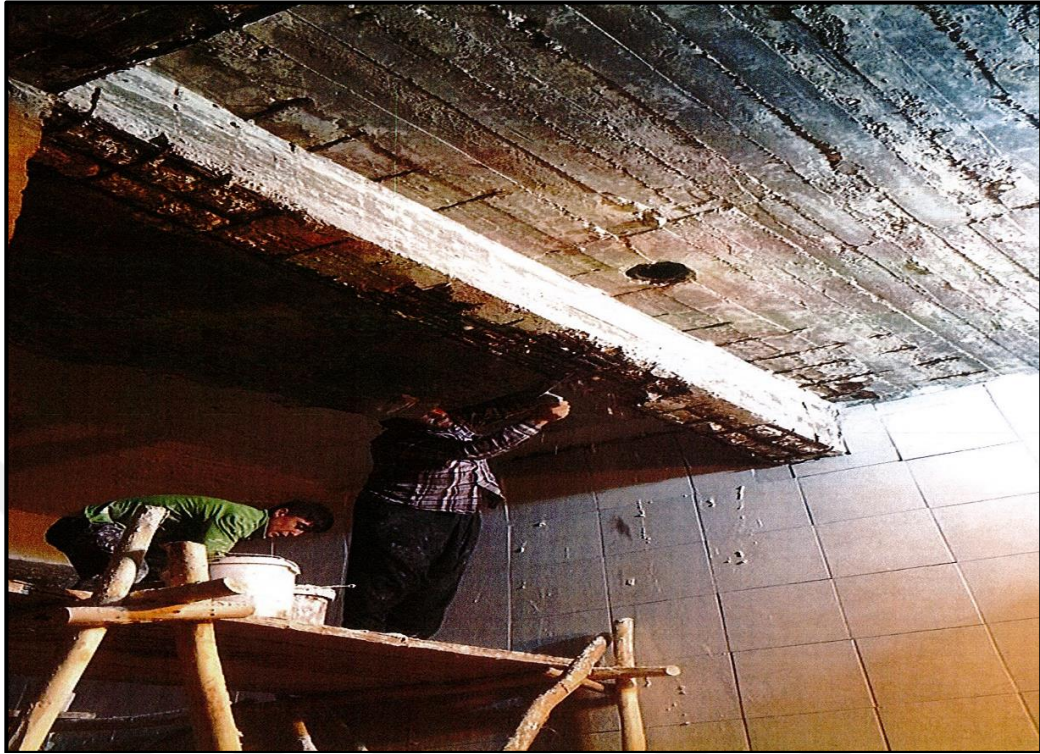
Figure A.1. Renewal of Water Storage Tanks
