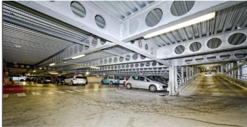
Figure 1. Parking structure (Arcelormittal, 2020a)
