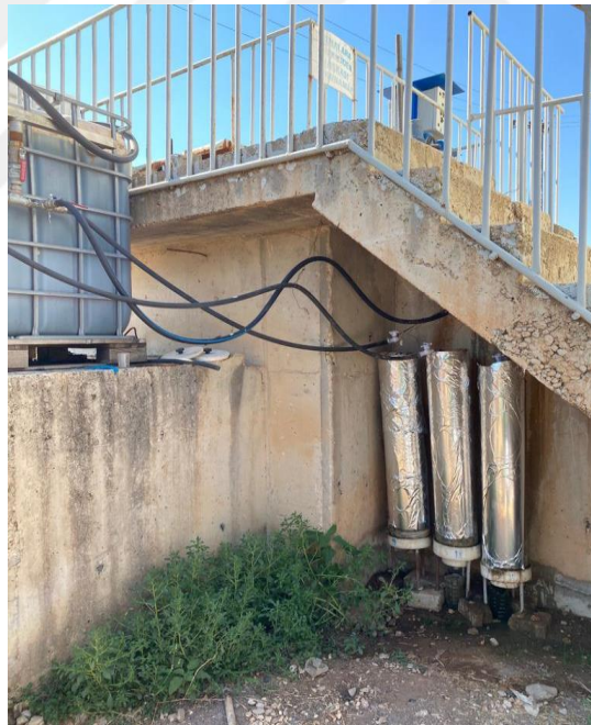
Figure 3.9 Feeding soil columns with wastewater after the second sedimentation.
