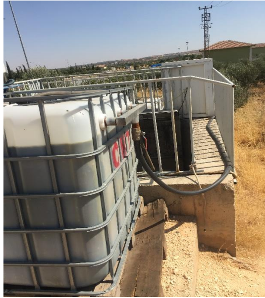
Figure 3.8 Wastewater passage from the first sedimentation tank to the second sedimentation tank.
