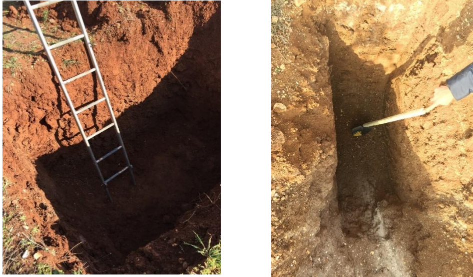
Figure 3.1 Excavation of soil samples.
