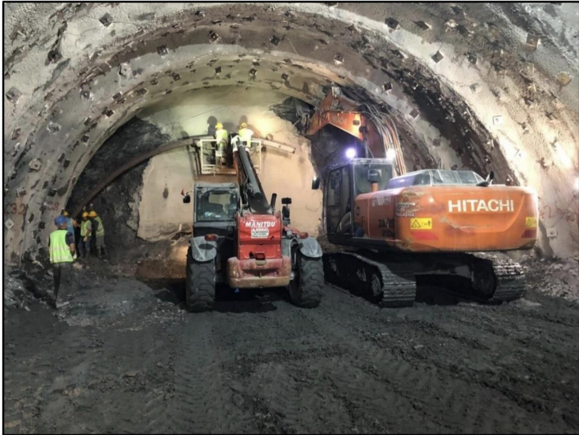
Figure 4.4. Upper half support installation of the tunnel.
