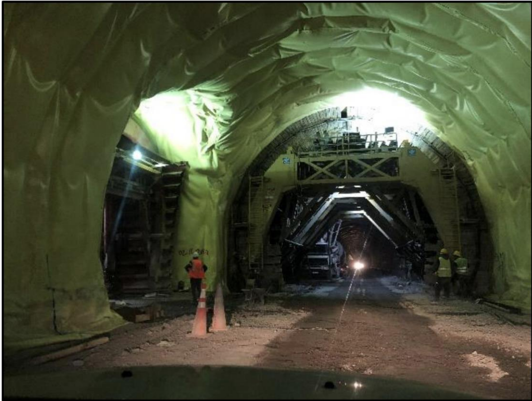
Figure 4.8. Application of geomembrane isolation in the tunnel.
