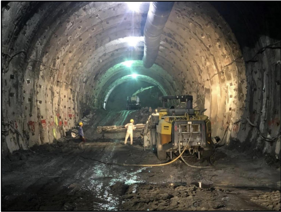
Figure 4.5. IBO bolt drilling and injections of the tunnel.
