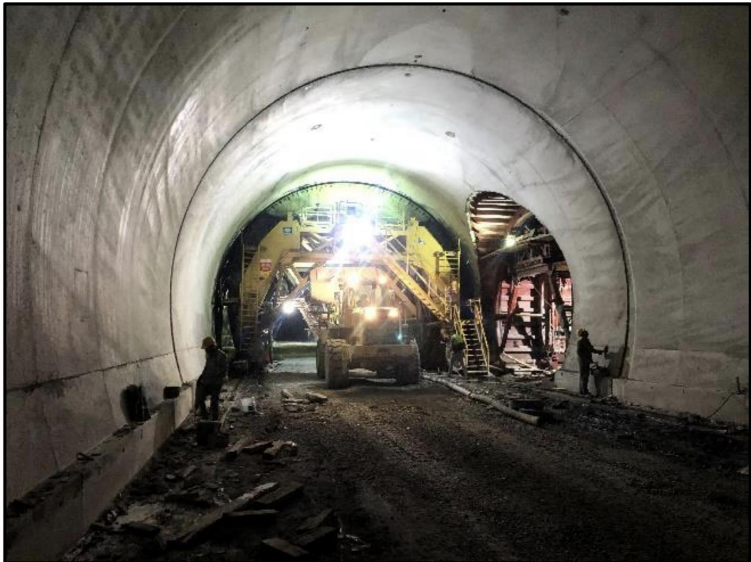
Figure 4.9. Concrete application inside the tunnel.
