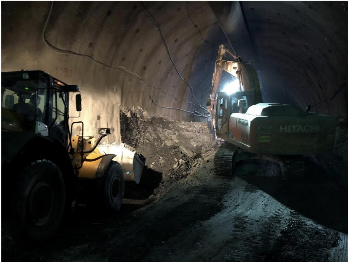
Figure 4.6. Bench excavation and waste transport.
