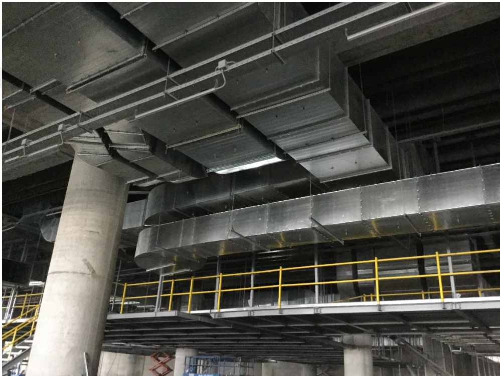
Figure 49: An example of BIM compatible site installation
