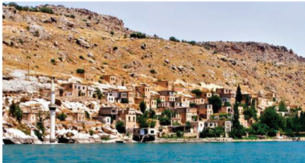
General view of the old Halfeti settlement
