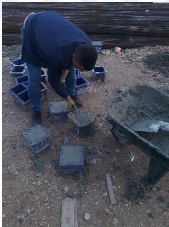
Figure 3.12 Getting The Mix In The Wheelbarrow
