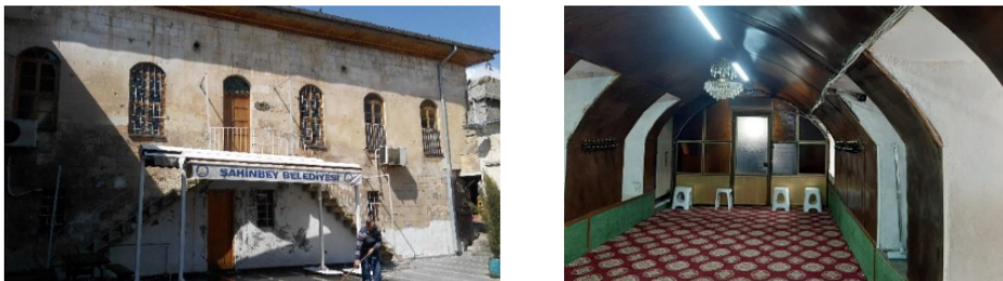
Image 11. Bekirbey Madrasah entrance facade (left) and interior view (right)
