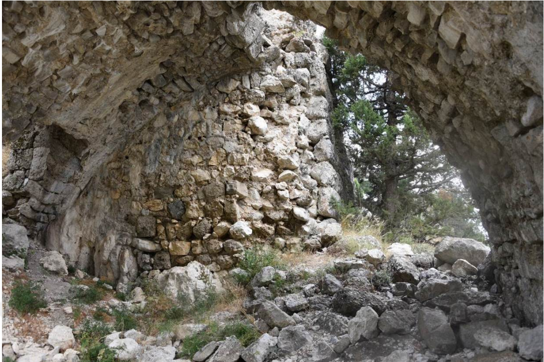
Figure 3.38: Structure B Space Z02
