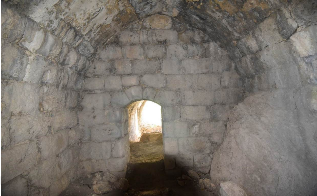
Figure 3.45: Structure C Space No. 202
