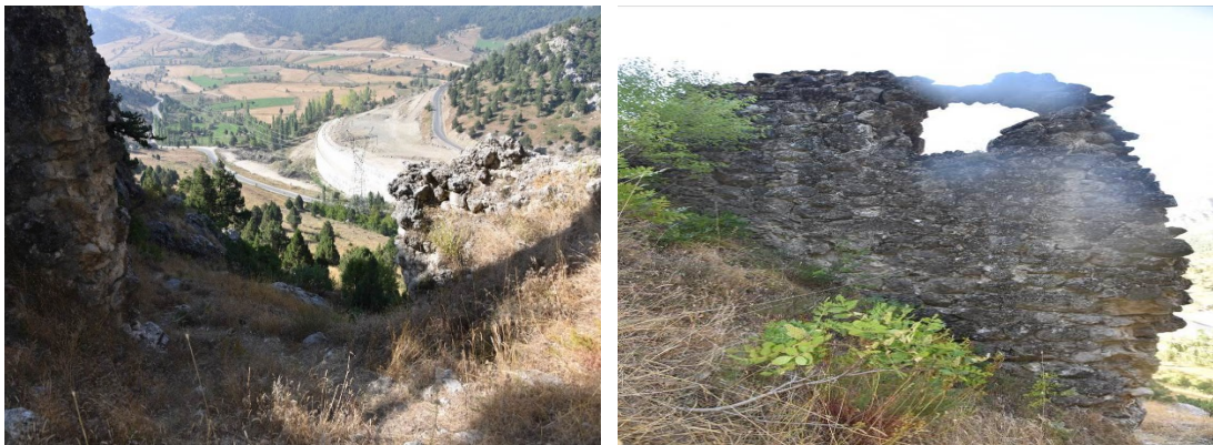
Figure 3.21: 1. Courtyard Inner Fortification Walls
