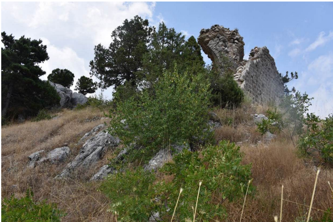
Figure 3.51: Structure D South Front
