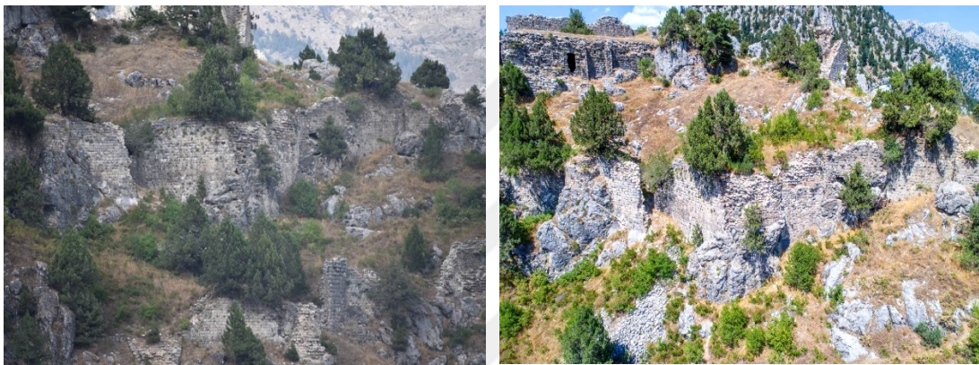
Figure 3.20: 1. Courtyard Inner Fortification Walls -2
