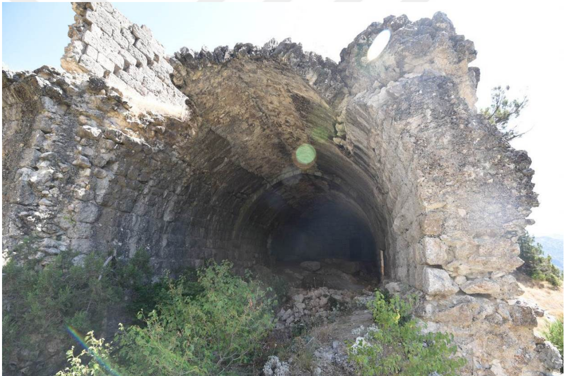
Figure 3.41: Structure C Western Front
