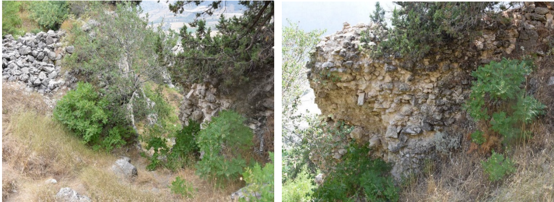
Figure 3.22: 2. Courtyard Inner Fortification Walls
