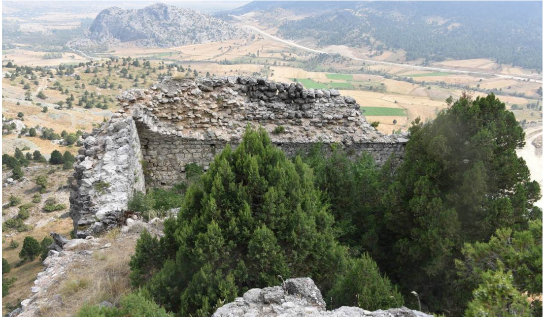
Figure 3.30: Structure A Northern Front
