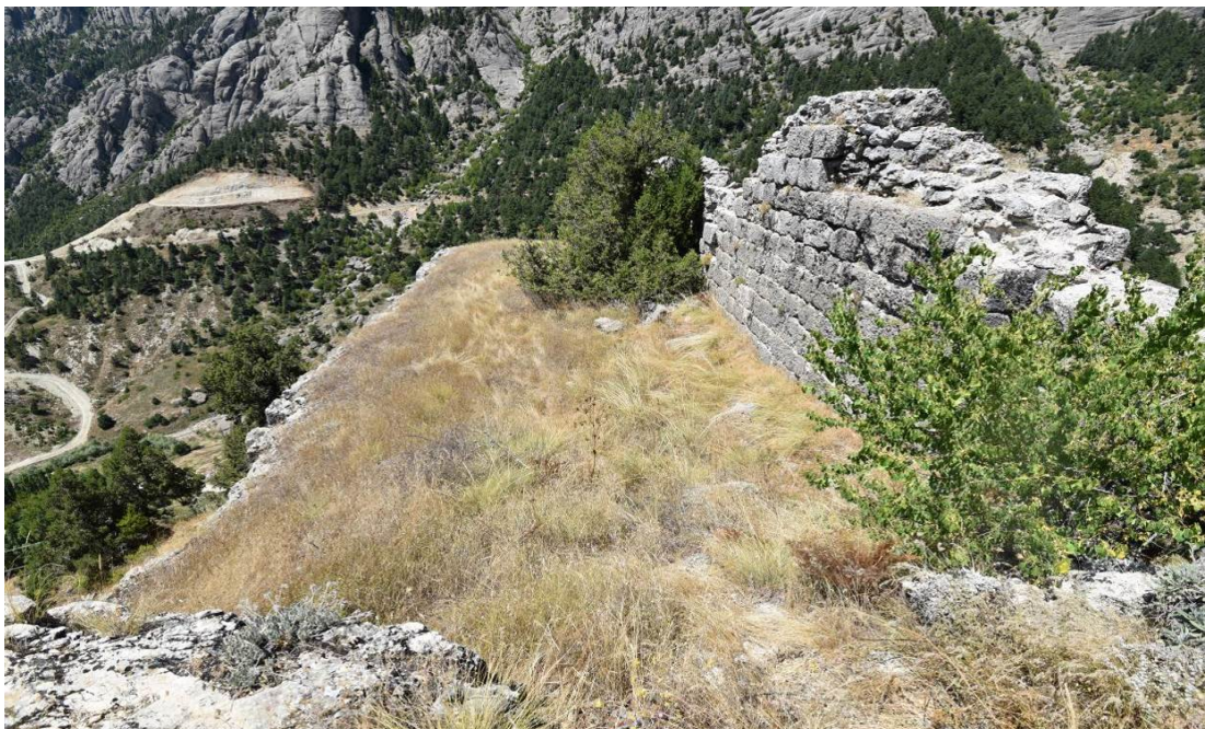
Figure 3.46: Structure C Space No. 301
