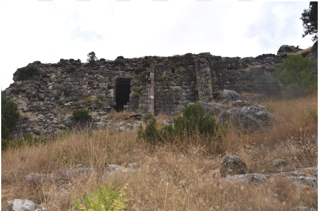
Figure 3.40: Structure C South Front
