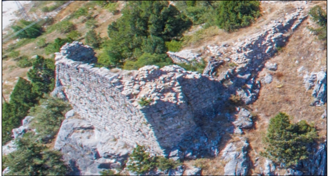
Figure 4.1: A Structure Drone Appearance
