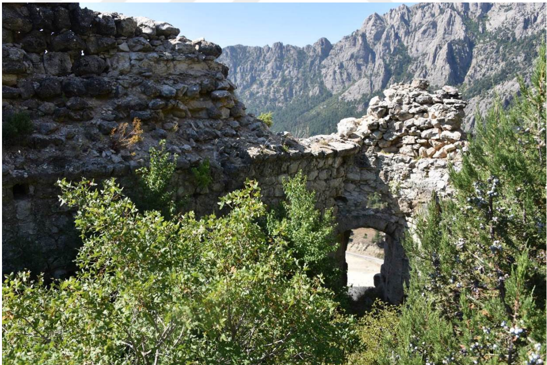
Figure 3.36: Structure A Space-2 Z01
