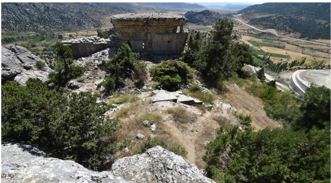
Figure 3.48: Structure D Overview
