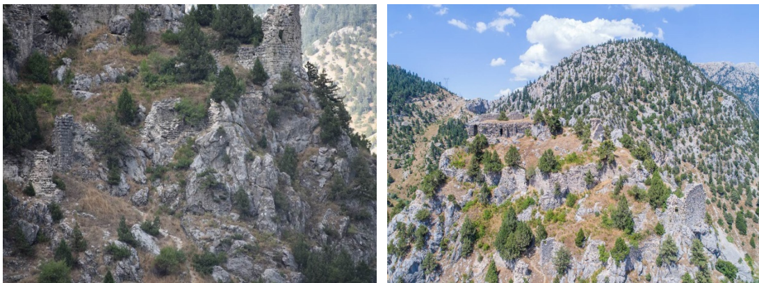
Figure 3.19: 1. Courtyard Inner Fortification Walls -1
