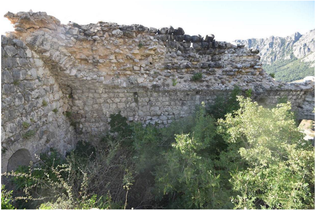
Figure 3.35: Structure A Space-1 Z01
