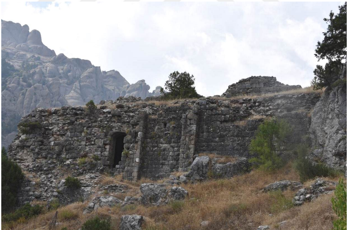
Figure 3.39: Structure C General Appearance
