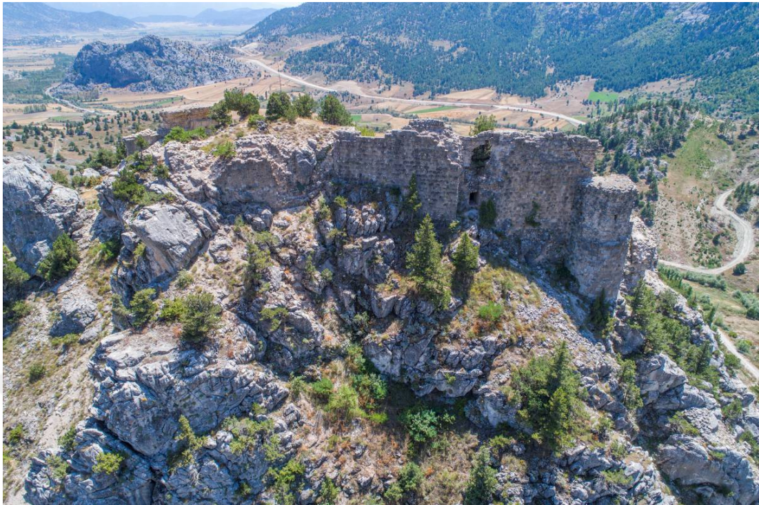
Figure 3.23: North Front General Appearance
