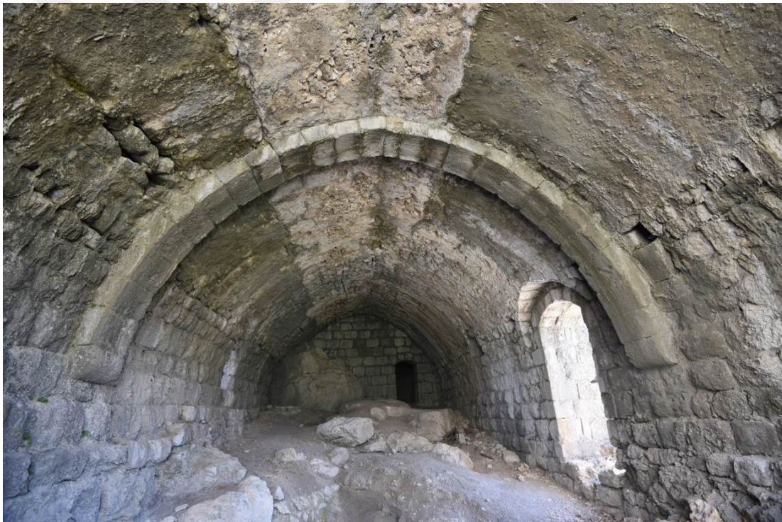
Figure 3.43: Structure C Space No. 201
