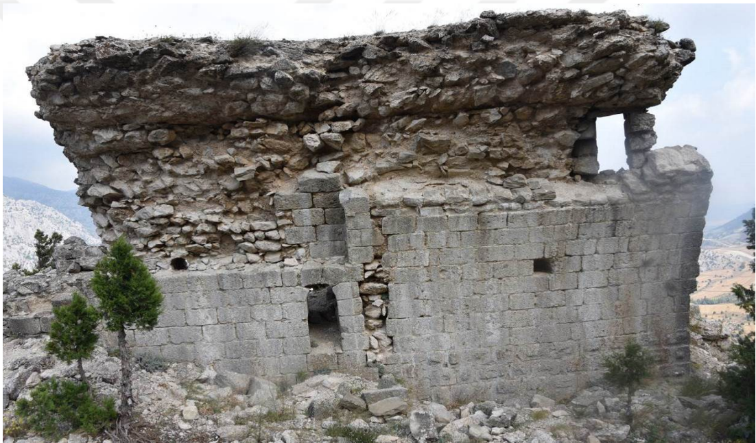
Figure 3.49: Structure D Western Front
