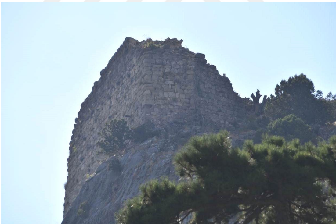
Figure 3.29: Structure A General Appearance
