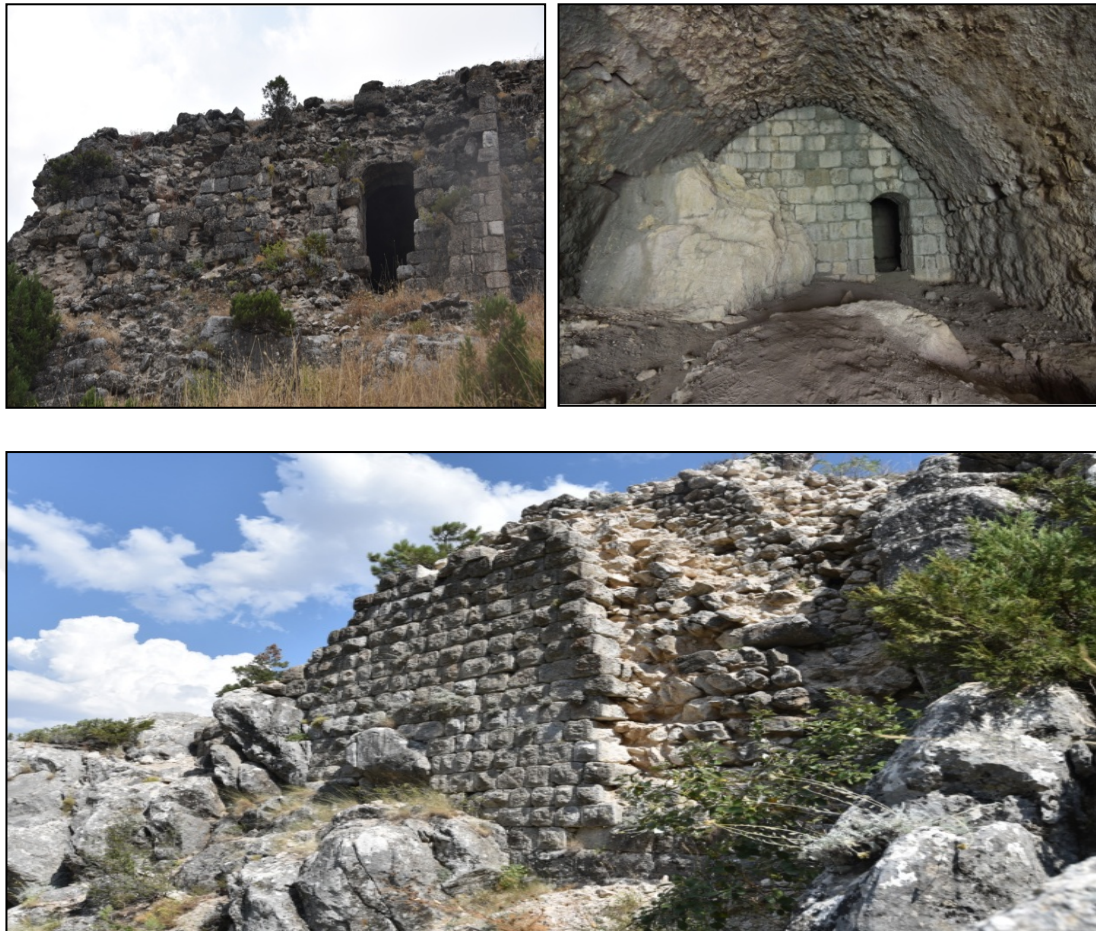
Figure 4.3: Structure of C; a) Southern Front rundown buttresses and semi-rundown 3. Strut view b) Main flat vault space. c) Vault Exterior North Facade Wall Losses
