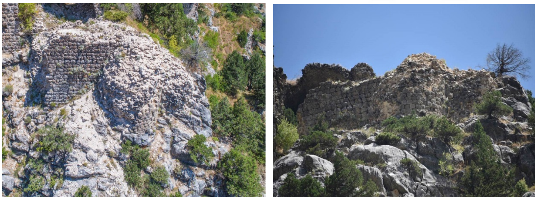
Figure 3.28: 2. Courtyard Exterior Fortification walls
