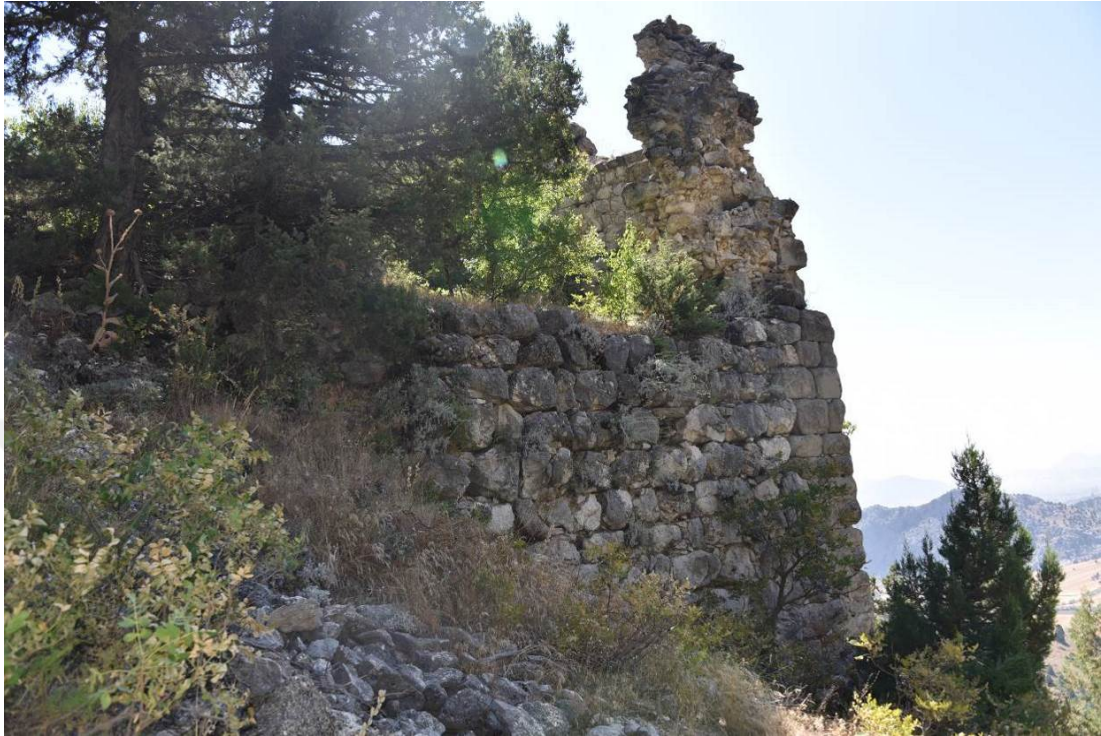
Figure 3.34: Structure A Southwest Front
