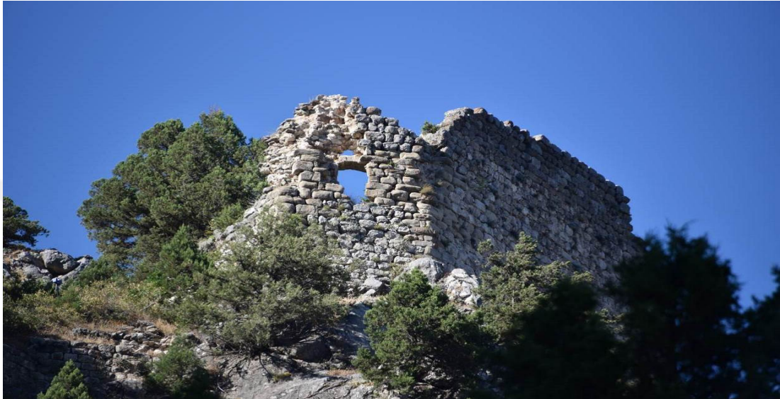
Figure 3.32: Structure A Southern Front
