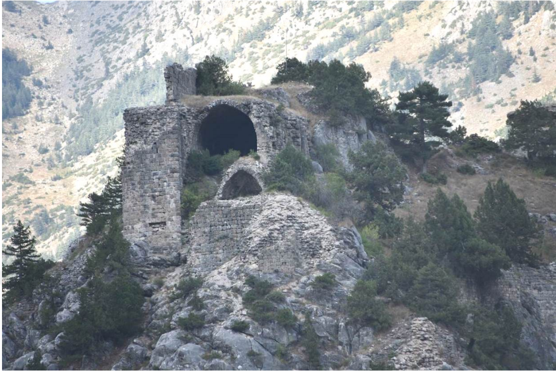
Figure 3.37: Building B General Appearance
