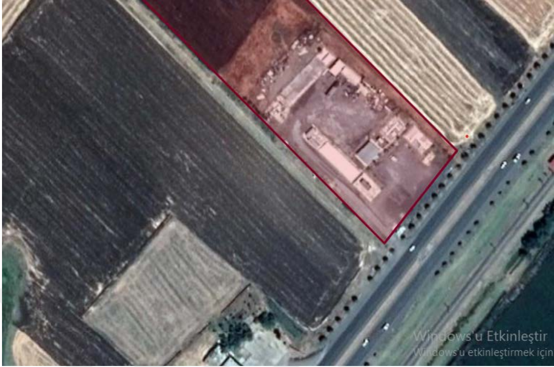
Figure 3.2 Area of testing
