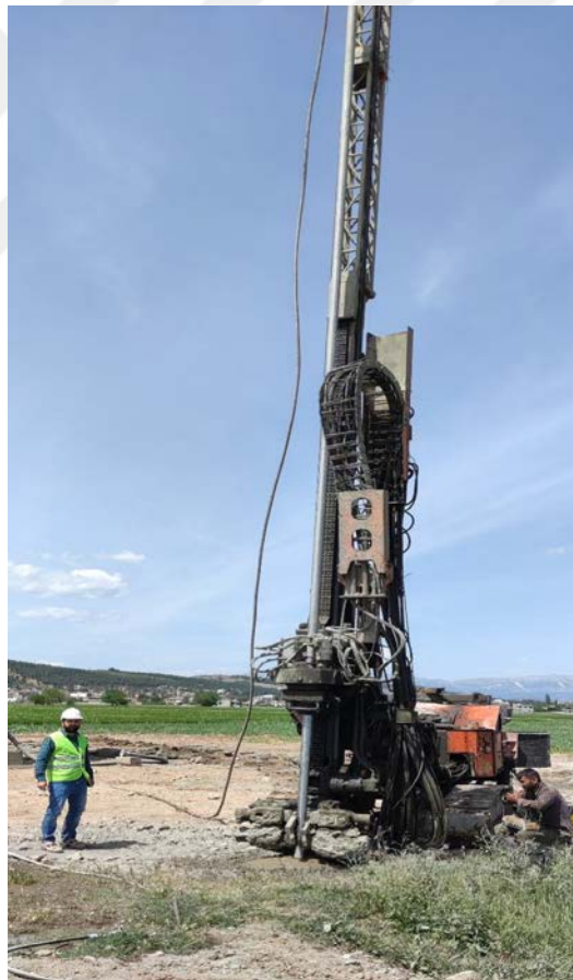
Figure 3.3 Jet grout testing machine
