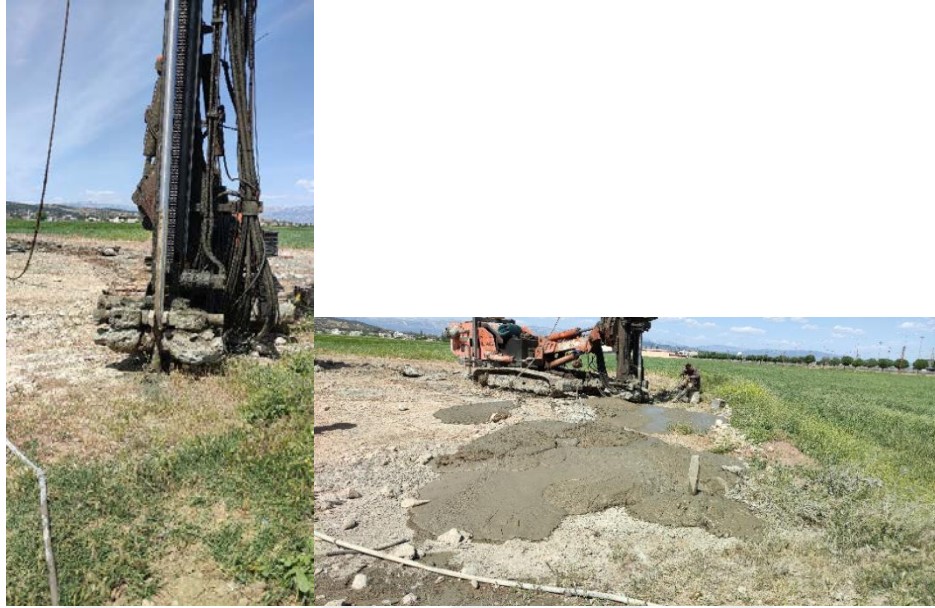
Figure 4.1 JG column production stages
