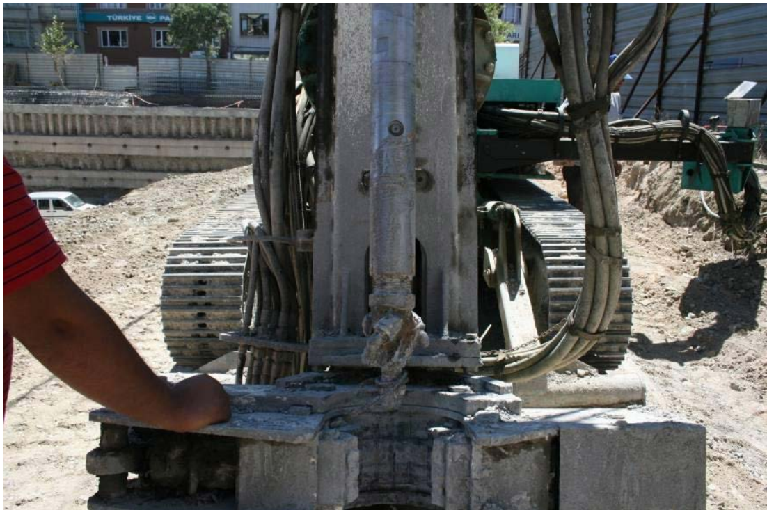
Figure 2.13 Drill pit for jet grout column production.
