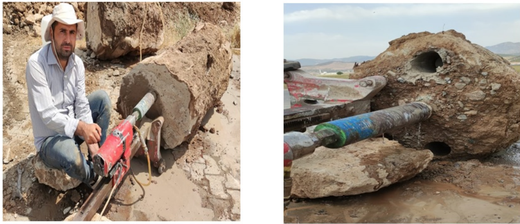
Figure 4.9 Taking core samples of JG columns
