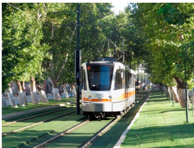
Fig. 3. The artificial green grass on the route of the tramway (World Trams and Traleibus Systems, ymtram.mashke.org , 2013). (For interpretation of the references to colour in this figure legend, the reader is referred to the Web version of this article.)
