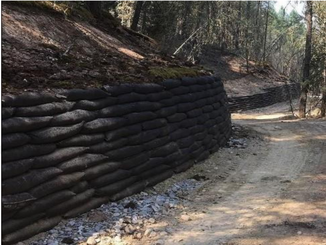
Figure 1.2 MSE wall with sloping backfill
