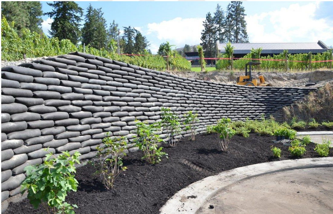
Figure 1.1 MSE wall example (Wall System, 2021)
