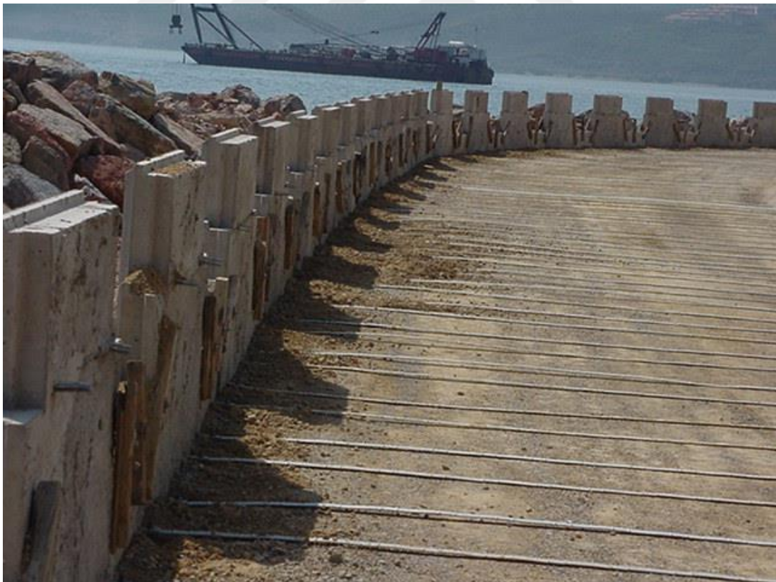
Figure 1.3 Steel strip reinforcement (Reinforced Earth, 2019)
