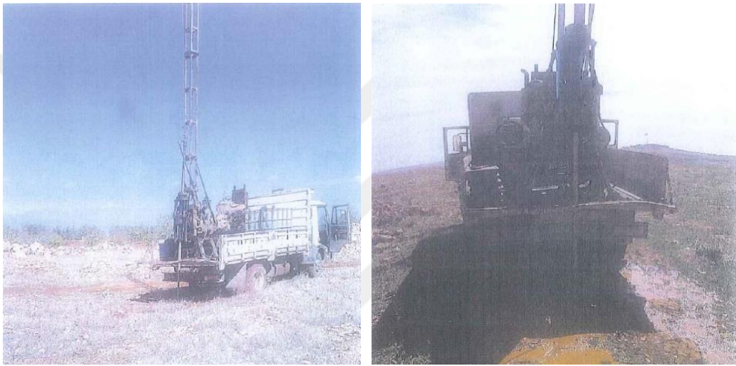
Figure 3. 1 Soil and foundation investigation
