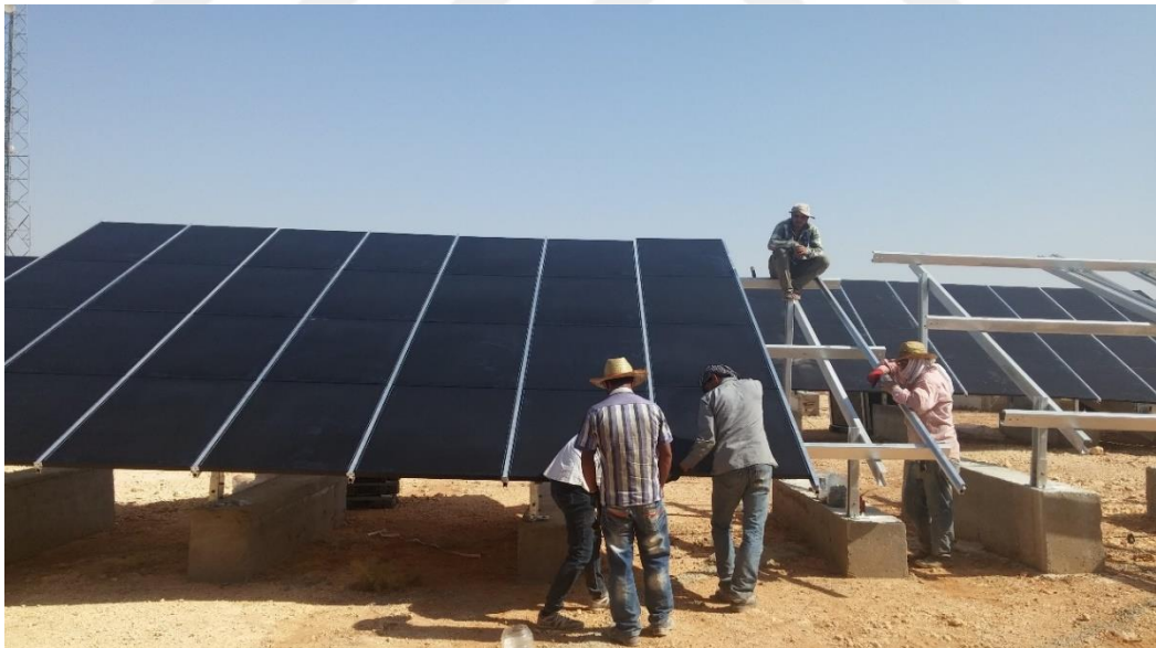
Figure 3. 7 The installation of modules
