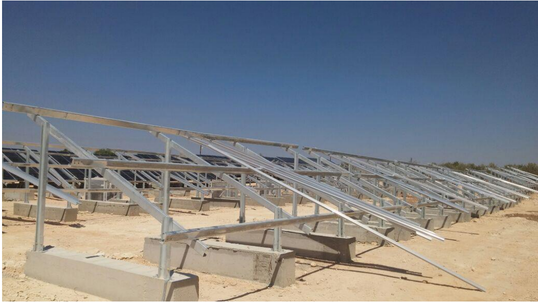
Figure 3. 6 An image of steel carrier construction
