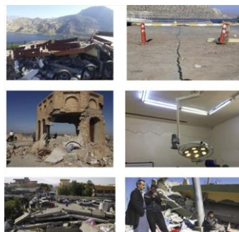
Figure 2.1 Damages to various structures in Iraq as a result of the Halabjah
