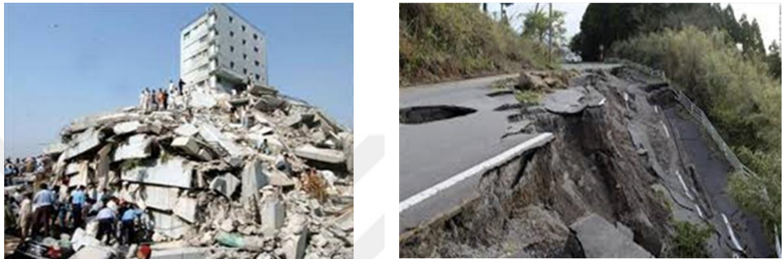
Figure 2.3 Damages of Lebanon earthquake
